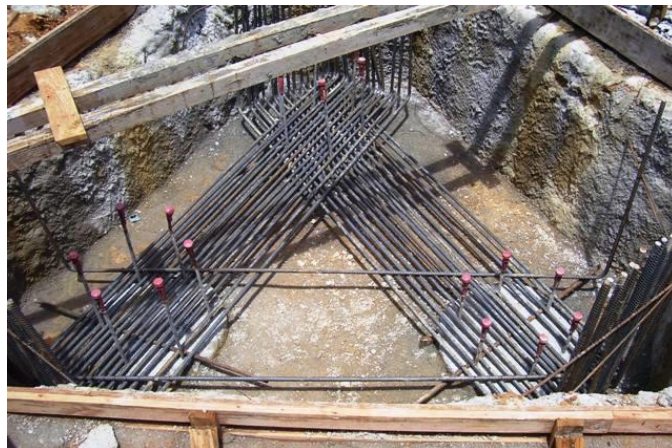
Figura 16: armadura principal in loco
